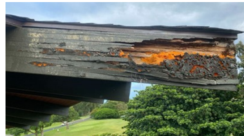
Exterior Wood Repairs (Lanai Decks/Beams)
